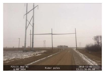
Wooden rider poles are a safety catch for the conductor (power line) as its being strung from structure to structure across the highway. The poles sit well above the road to ensure that there is no chance of the conductor contacting the roadway or vehicles on it. [pictured above]
